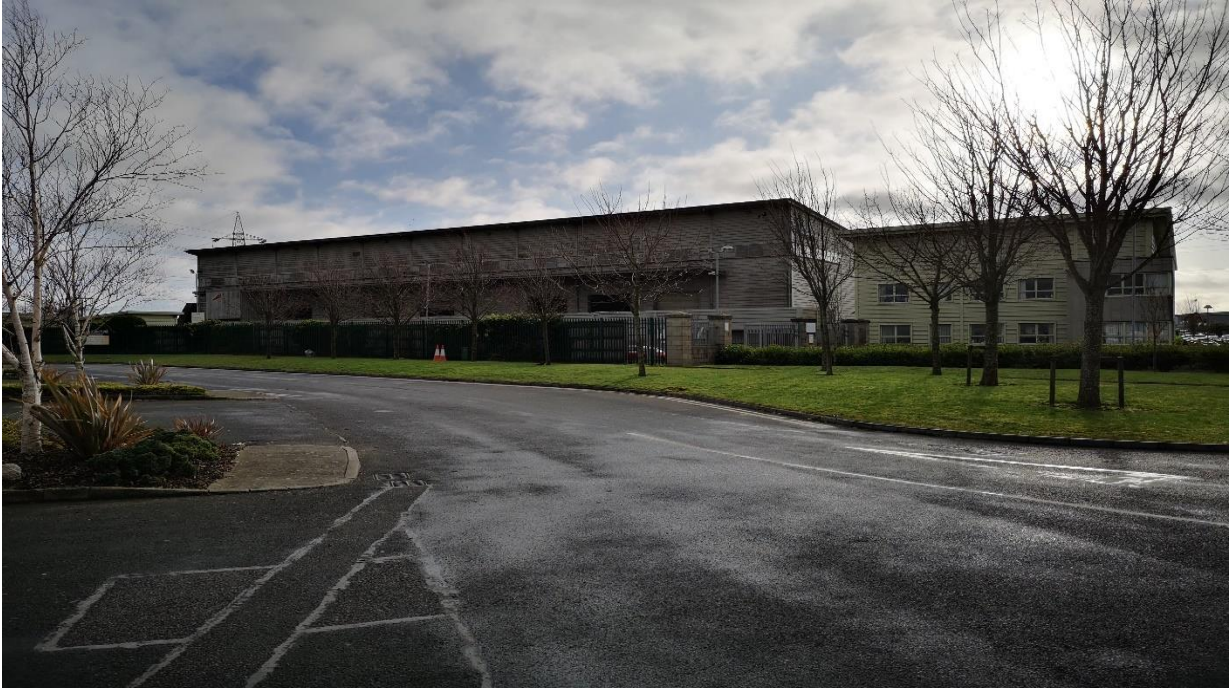
Photograph 12.1 View of Office and MP1 & MP2 from North West
