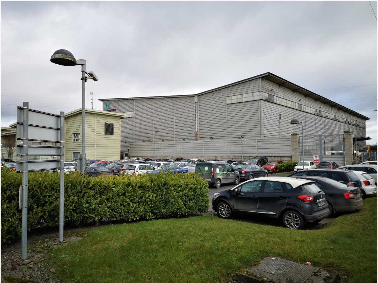
Photograph 12.3 View of Eastern Elevation of MP1 & MP2 From Business Park
