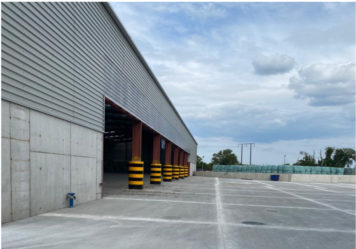
Photograph 12.8 Internal View of Southern Elevation of MP3 & External Storage Area
