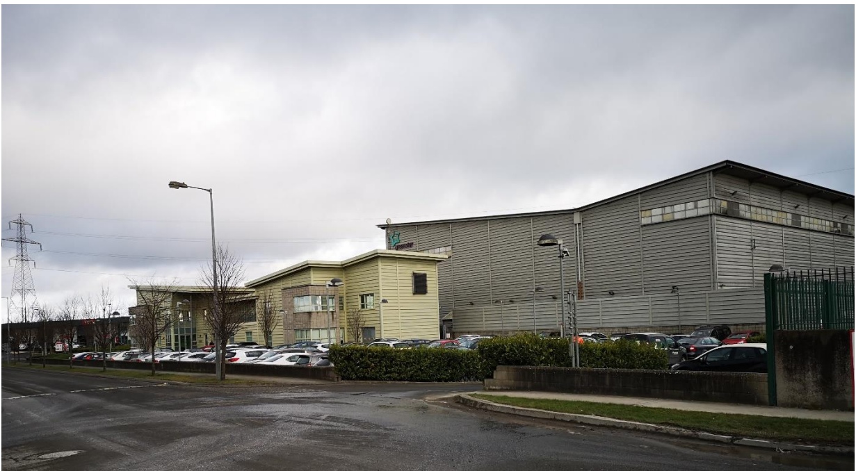
Photograph 12.2 View of Office and MP1 & MP2 from South
