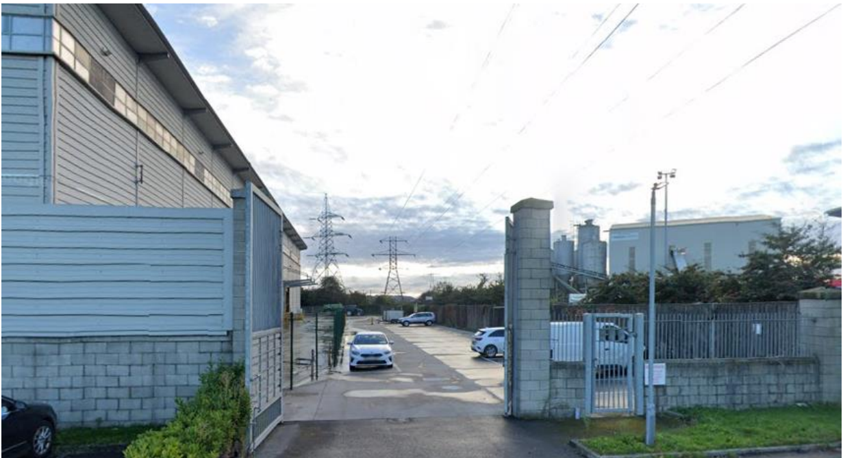
Photograph 12.4 View From Car Park Looking East (Concrete Plant on Right)
