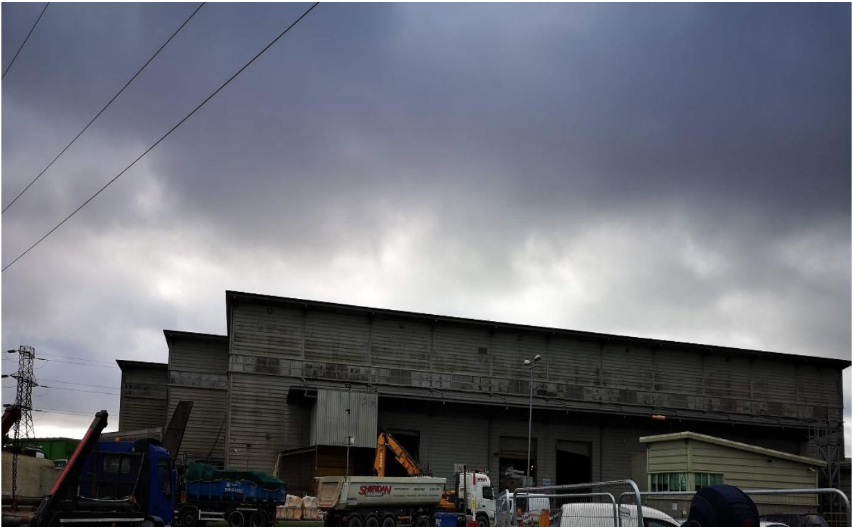
Photograph 12.6 Internal View of Northern Elevation of MP1 & MP2
